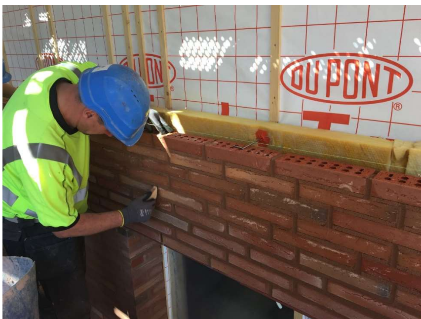
Murarbeid for Munch Brygge i felt B4.
